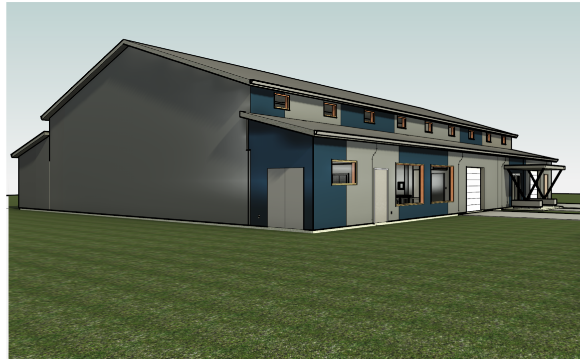
3 Exterior - South East
