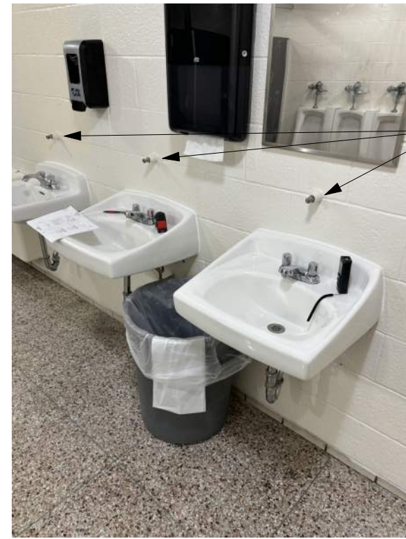
PROTRUDING ELEMENTS TO BE REMOVED IN RESTROOMS A114 & A115
