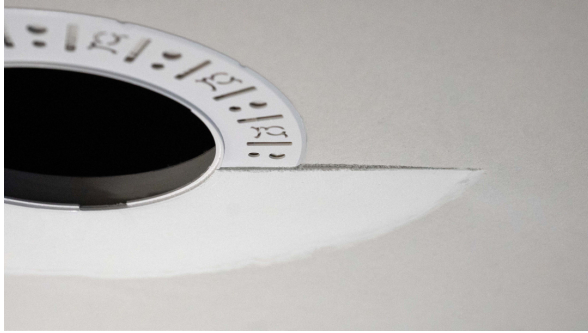
Partially finished mud ring, showing cross-section detail.
