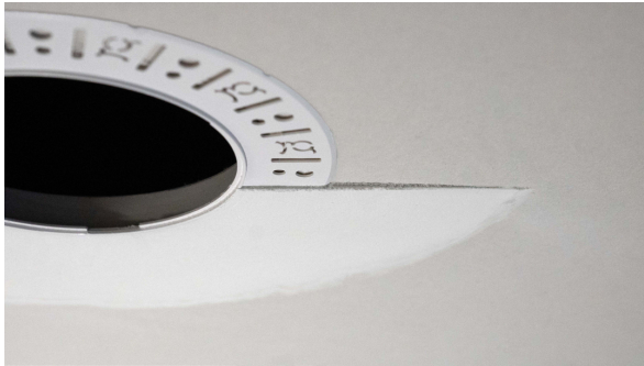
Partially finished mud ring, showing cross-section detail.
